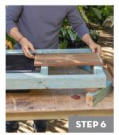
the predrilled assembly holes, predrill into frame beneath, then insert and tighten decking screws. Predrill 6 additional equally spaced holes into Long strip, and in line with screws on adjacent Short and middle strips. Insert and tighten decking screws.
