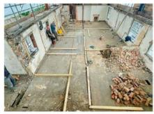
With the roof gone and the internal walls removed, timbers mark out positions of the landing and rooms on the first floor.
