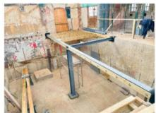
To gain more ceiling height, floors and ceilings were removed and repositioned, and space was absorbed from the loft.
