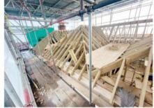
The builders rebuilt the three roof valleys at the back of the house to match the design of the original structure.
