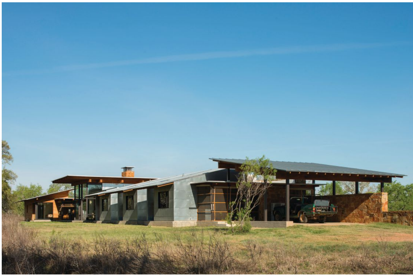
In total, approximately 5,000 square feet of face stone was employed for the home's design.
