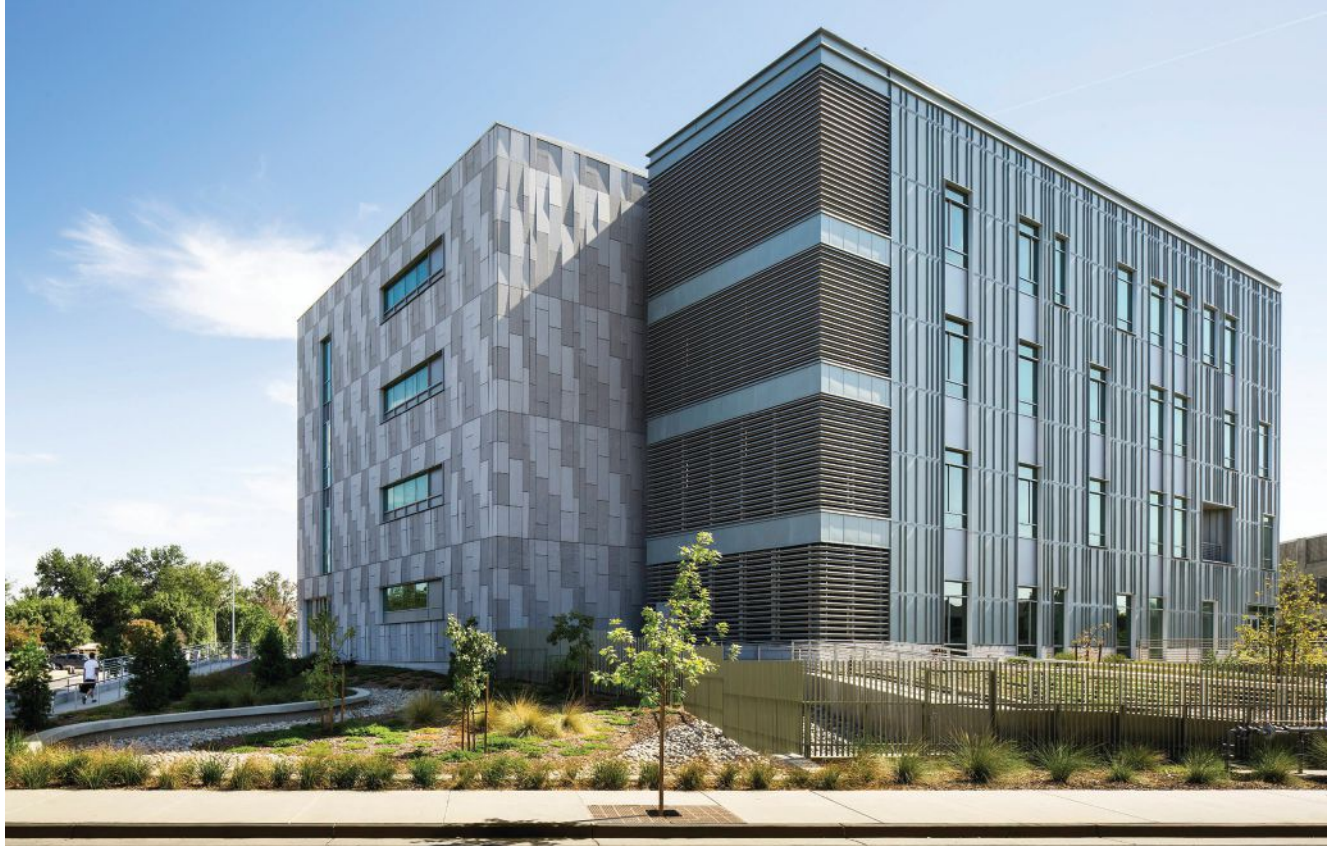
The exterior of the building boasts mechanically attached Sierra White™ granite in a vertical, basket-weave pattern.
